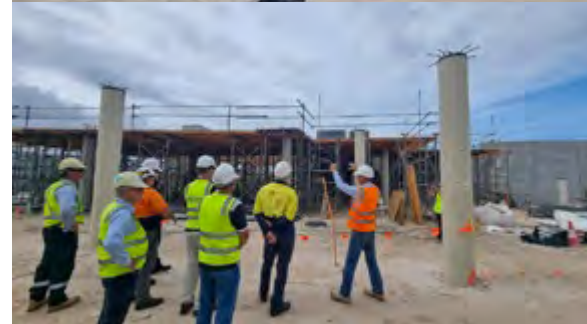
Byte Construct leads a tour of the new buildings in late 2024.
