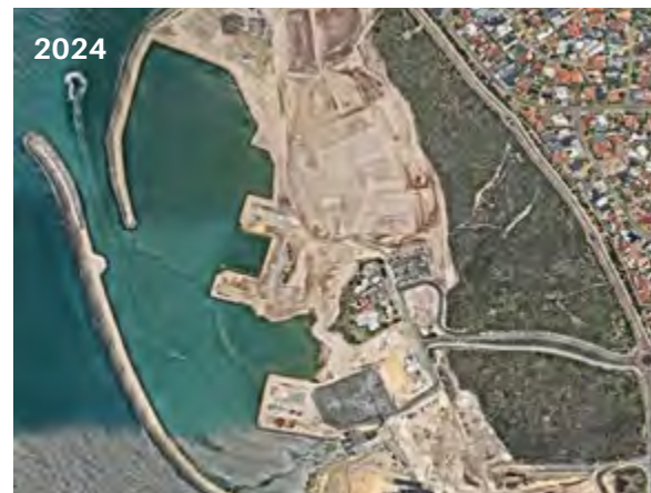
Take a look at the transformation - with the old marina boat harbour (top) and the current marina (bottom).
